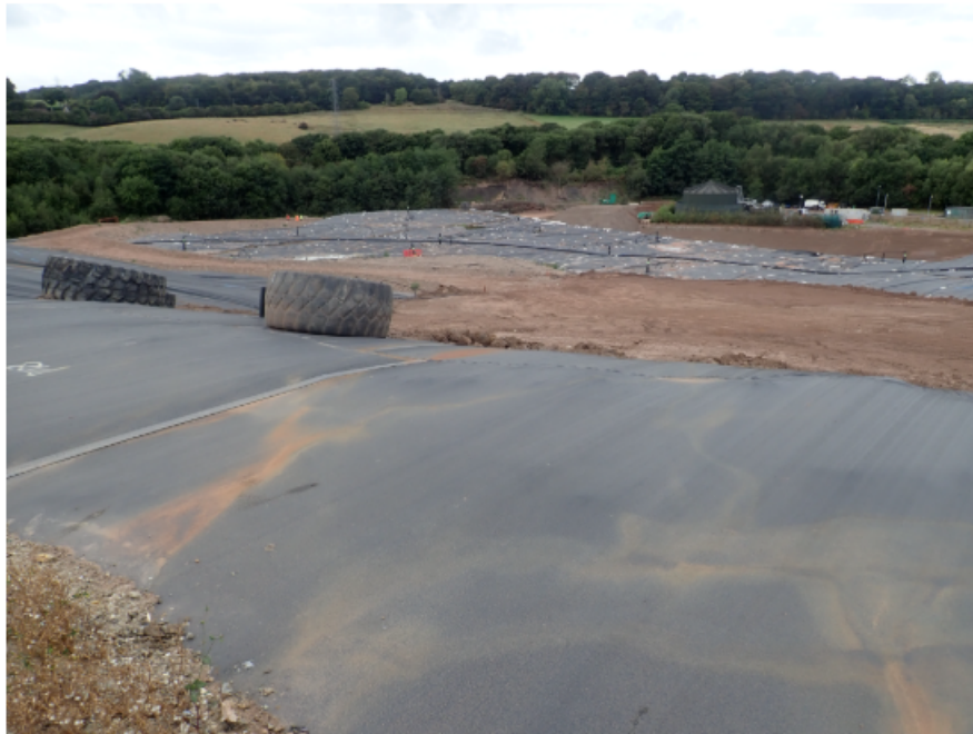
Photograph of depression work at the top of the site on 27 August 2025
