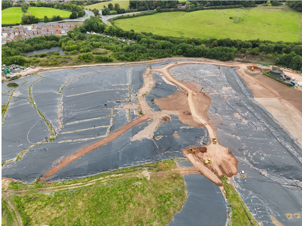
Photograph taken on 26 September 2025 showing clay placed on the site to remove the risk of fugitive landfill gas emissions
