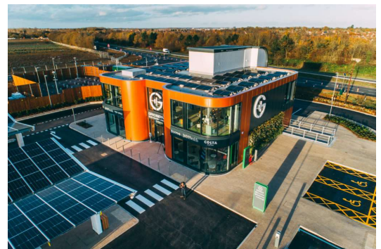
Figure 38: GRIDVOLT charging hub
