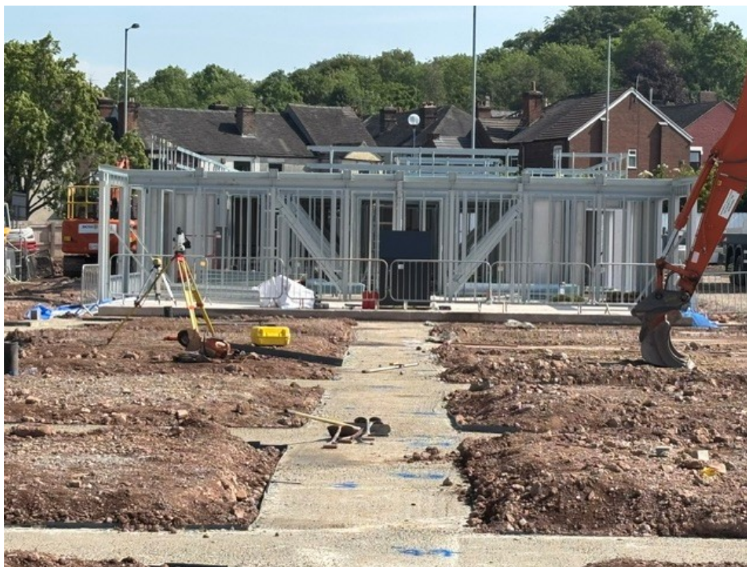
Central Apartment Block framing and foundations underway
