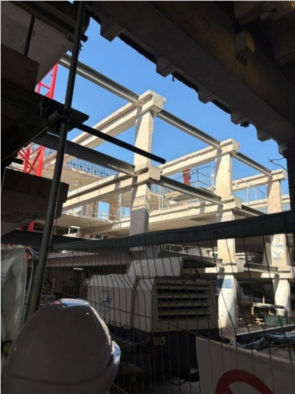
New Entrance created at undercroft with Boots / Roebuck
