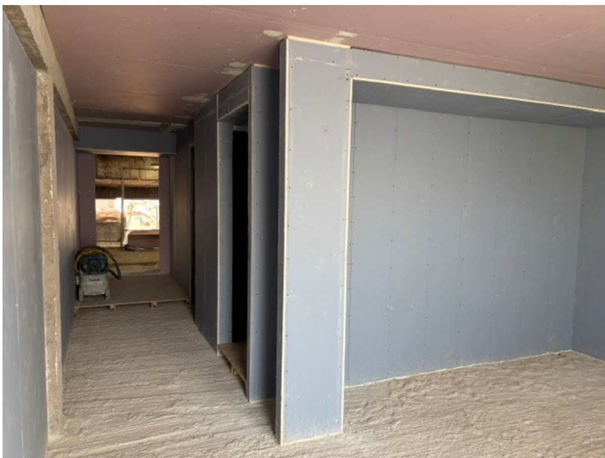
Internal wall fit out for apartments
