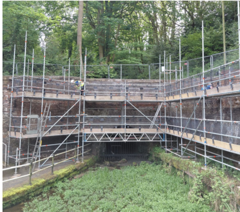
Works at Harecastle Tunnel
