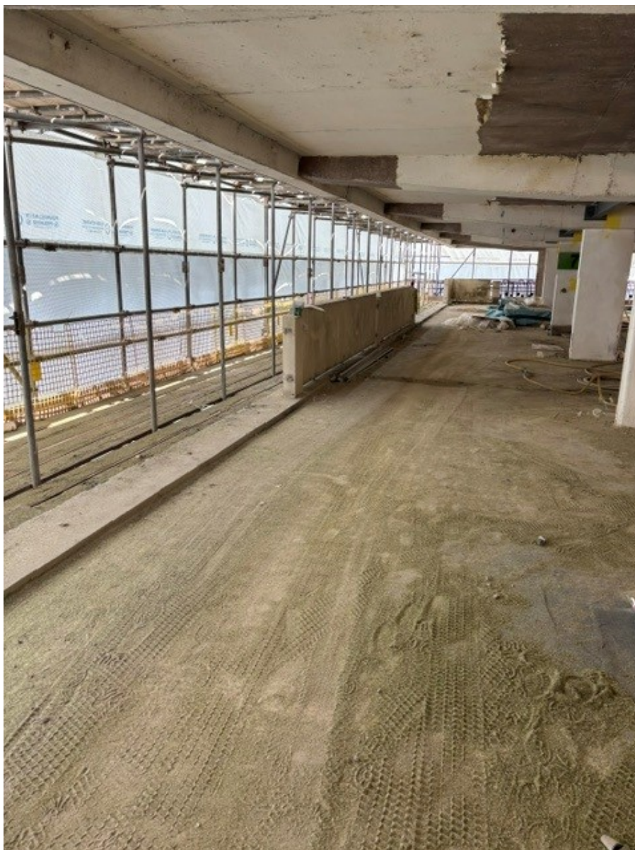
New Balustrade punch outs for apartment balcony
